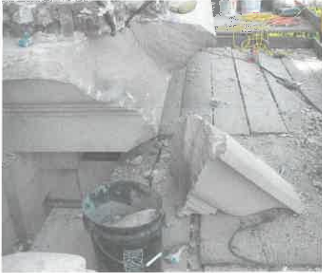
Portions of the limestone cornice were damaged to the point that they fell when work was being conducted and had to be pinned back in place.
